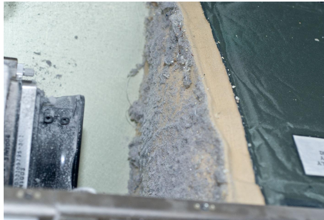
Ducting collects more dust than expected.
